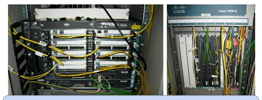
**Computers specialised for forwarding packets.** Different sizes and configurations depending on requirements.
